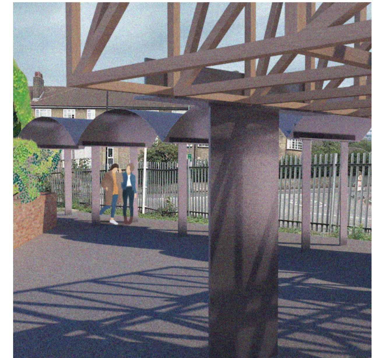
The corners of the trussed roofs cantilever from the centrally supported columns. The vaulted edge can be used as an extended entrance enfilade or subdivided to form individual vaulted spaces.
