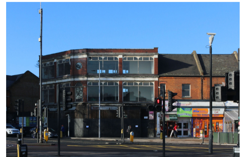
The elegant corner building has been left vacant since the 1980s
