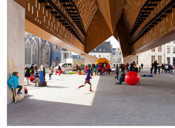
The Ghent Market Hall by Robbrecht & Daem and Marie Jose Vane Hee, is a covered space that forms no specific function but becomes inhabited through flexible community use.
